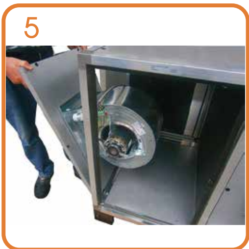
Invertire i 2 pannelli e collegare i fili del ventilatore Swap the two panels and connect the wires of the fan
